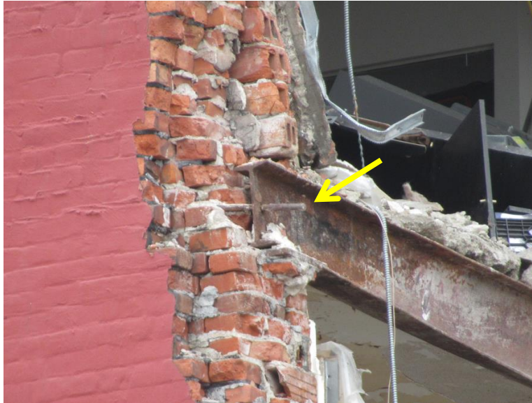
Fig. 3. Image taken by SEI on June 4, 2023, indicating beam pin (yellow arrow).
