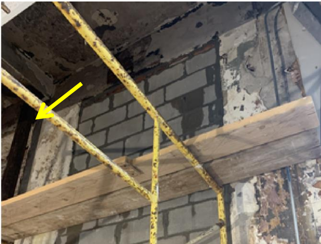
Photograph indicates inside of building with CMU installed inside window opening. Note shore previously identified at Pier D (yellow arrow).
