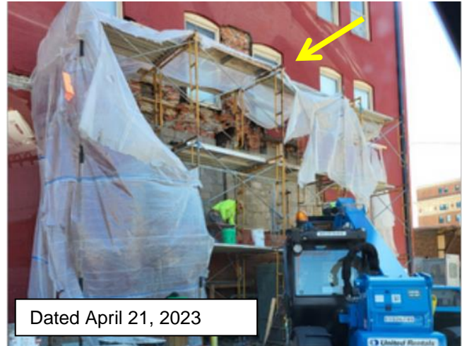
Overall view of repairs underway at southern end of west façade.
