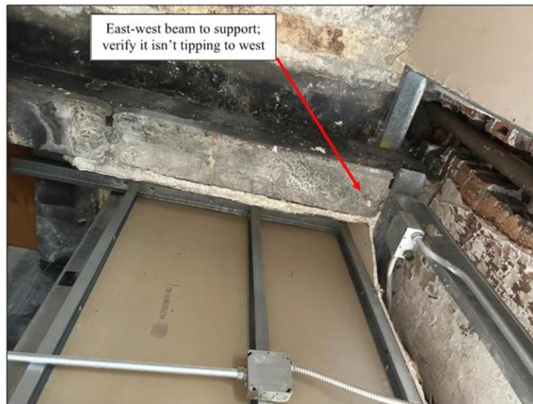
Photo 4 – Existing Beam to Support
