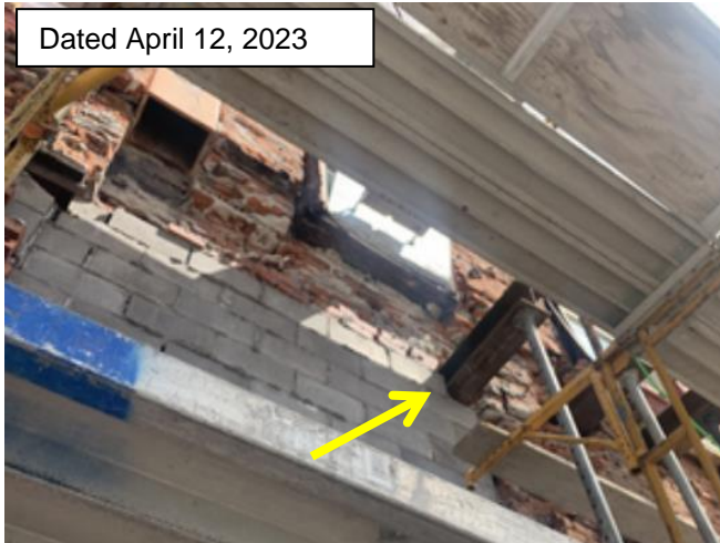
Photograph indicates repairs underway with use of needling beams evident.
