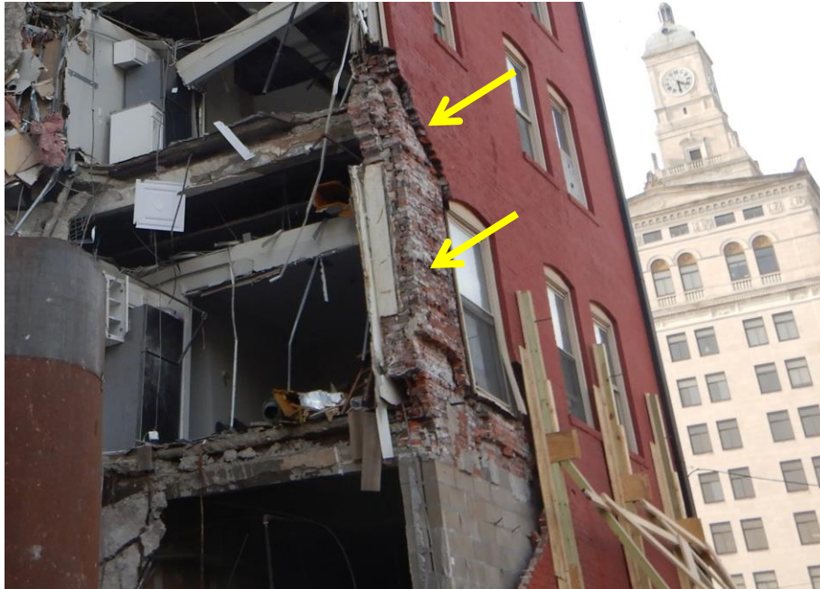
Photograph 19: Post-collapse view at wall cross section. Note outer 2 wythes of brick masonry not bearing on CMU replacement wall.
