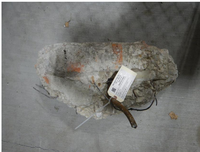
Appendix D – Photograph 4: Exemplar concrete floor slab material.
