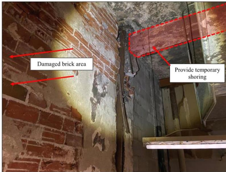
Photo 2 – Second Beam to Support
