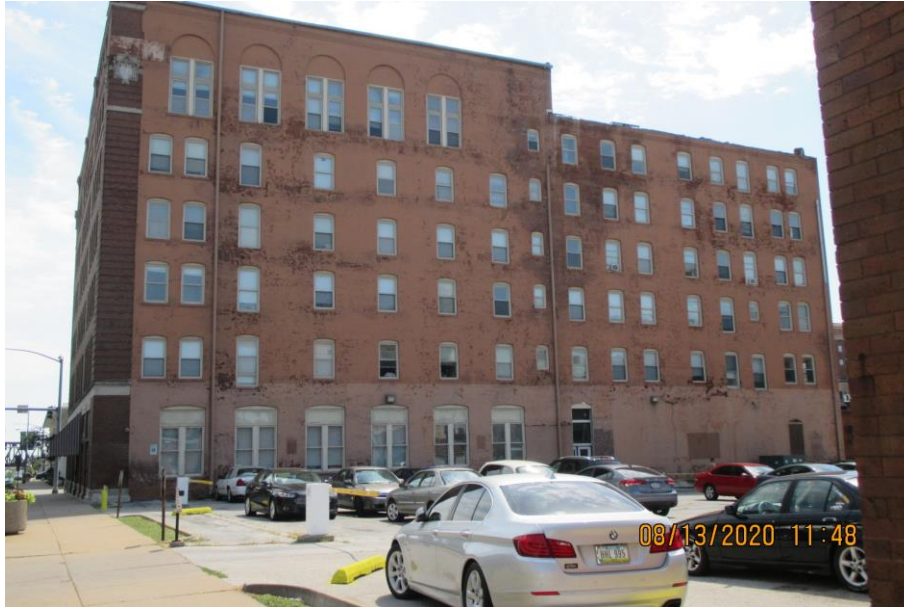
Photograph 1: August 2020 Image of west elevation from City report.
