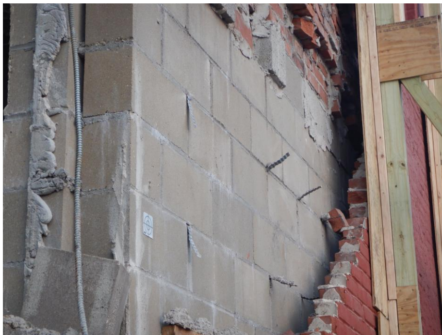
Photograph 20: Post-collapse image of CMU wall constructed in May 2023. Note corrugated brick ties not engaging outer wythe of brick masonry.
