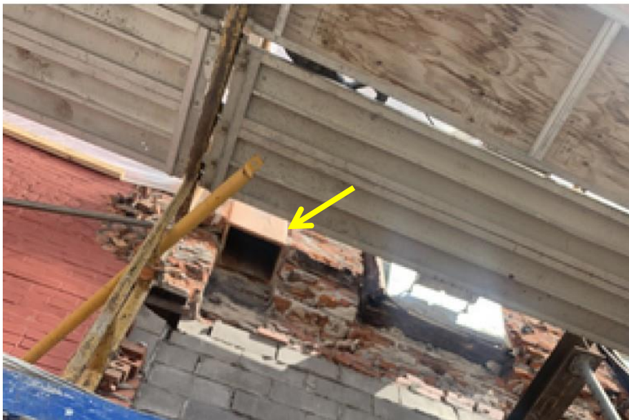
Photograph 26: Image from City file 23-9778 exhibiting April 2023 repair work. Note large vertical chase embedded within wall at Pier F.
