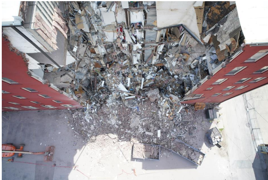
Photograph 36: Post collapse aerial image of subject Building from Shive Hattery sUAS.
