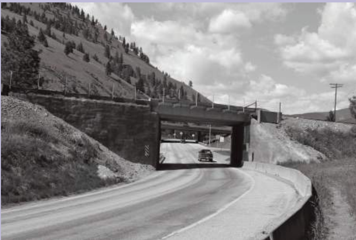
Existing Railroad Bridge
