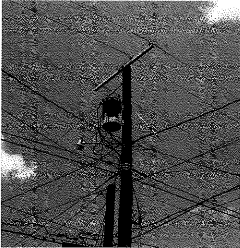
Figure 2: Rusting Transformer
